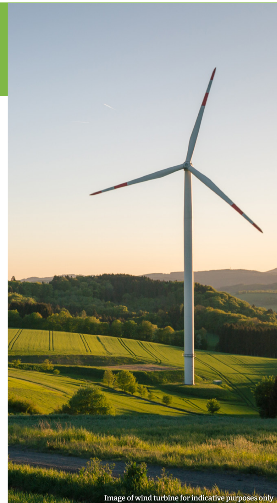
Image of wind turbine for indicative purposes only
